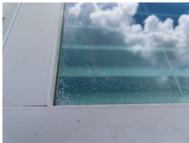
7.7 Item 4 (Picture) Kitchen
