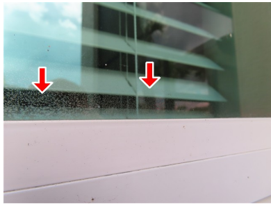
7.7 Item 1 (Picture) Office window
