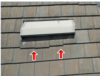
1.5 Item 5 (Picture) Rear slope
