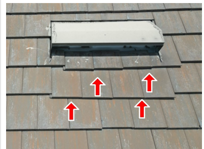
1.5 Item 7 (Picture) Left slope
