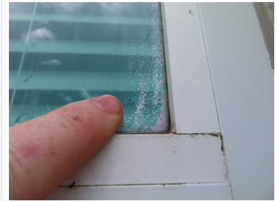
7.7 Item 3 (Picture) Kitchen
