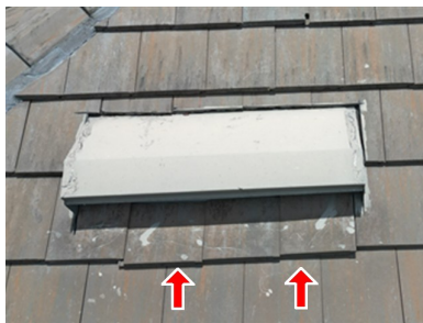
1.5 Item 6 (Picture) Rear slope
