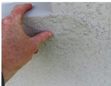
5.4 Item 2 (Picture) Left side
